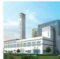
XUANWEI SECOND WASTE TO ENERGY PLANT
