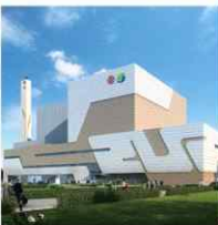
YUSHU WASTE TO ENERGY PLANT
